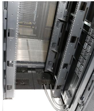
To ensure maximum protection against bypass airflow, each cabinet in the Fujitsu Services UK facility has been fitted with a KoldLok Extended Grommet accompanied by a heavy duty steel plate, custom-built by EDP.
